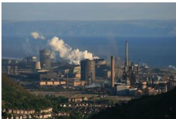
Tata Steel Works, Aberavon
